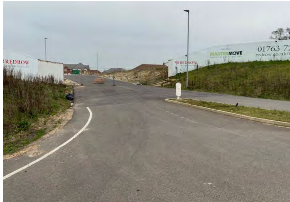
View from the new access point from the A10, looking east
