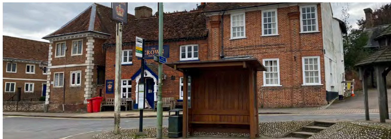
Bus stop along the High Street
